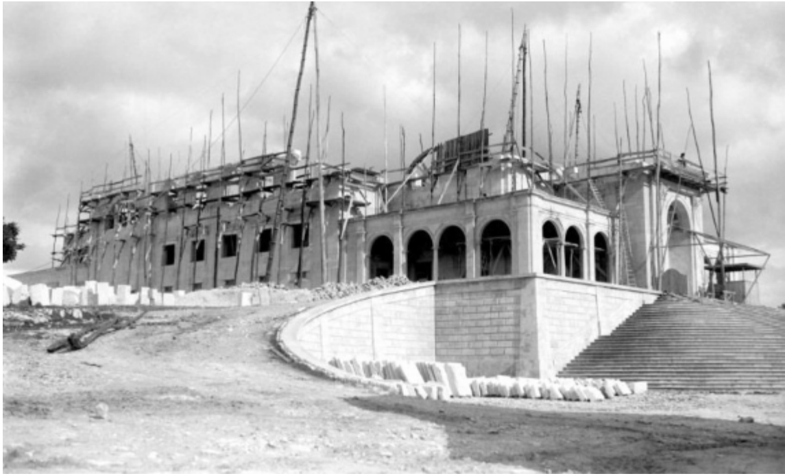
Anex 16. Initial phase of the construction of the church
