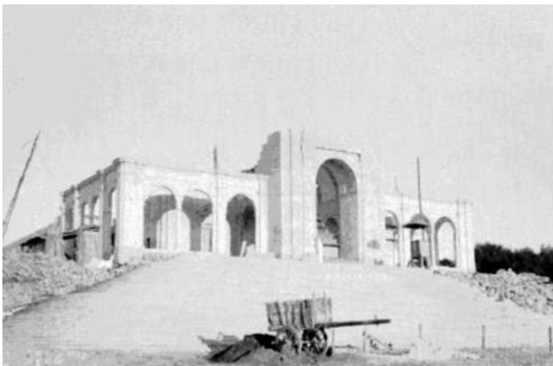
Anex 14. Initial phase of the construction of the church
